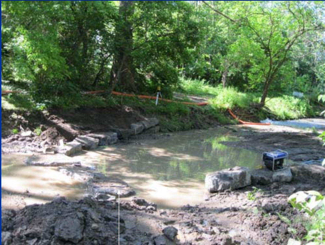
Partially installed Cross Vane
