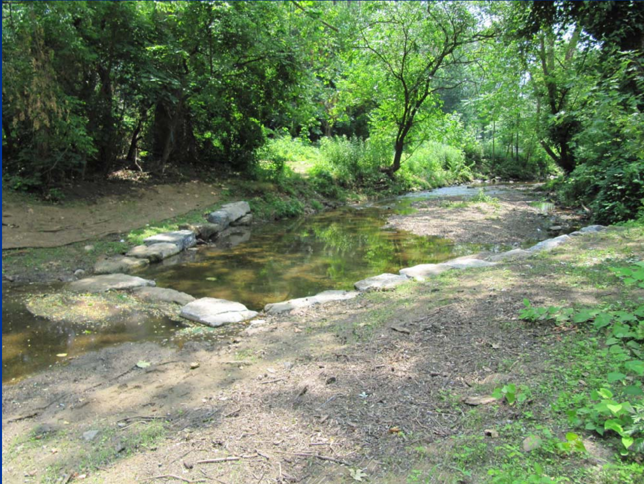
Little Crum Creek Cross Vane #1 after matting & seeding -viewed from above
